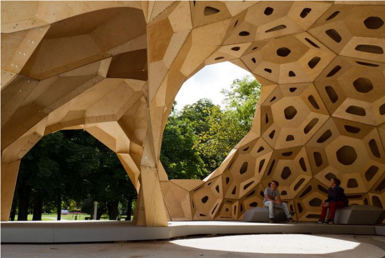
Research pavilion of robot-made segments, modeled on the sea urchin skeleton. Photo: ICD/ITKE (Institute for Computational Design / Institute of Building Structures and Structural Design, Stuttgart)
