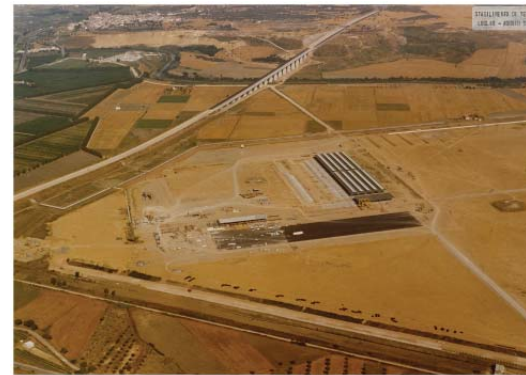
2. Fiat Factory of Termoli -Molise region- under construction (July-August 1972). Fiat Historical Archives, no box or folder.
