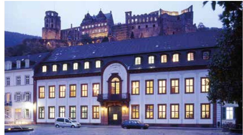
The headquarters of the Heidelberg Academy of Sciences and Humanities are located below Heidelberg Castle.
