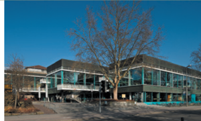
The cafeteria on Wilhelmstrasse is to be fully renovated
