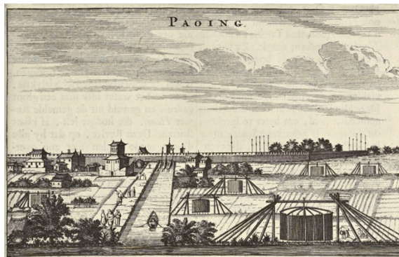
Figure 13: Vertical-axle windmills in Baoying 寶應 (Nieuhof 1665, image from p. 119 of the 1693 edition).
