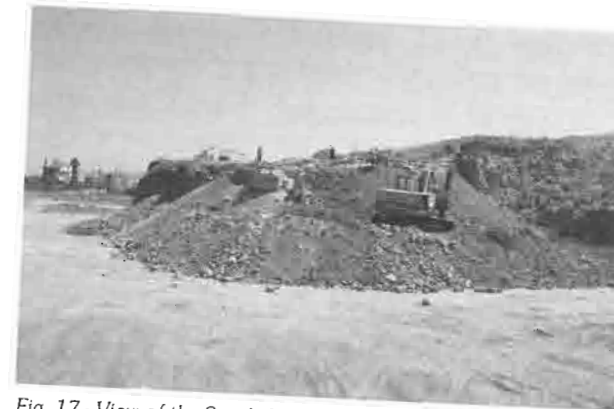
Fig. 17 - View of the South Section during the backfilling process.
