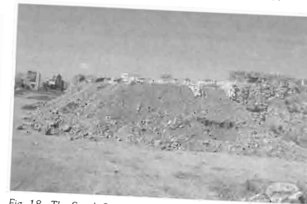
Fig. 18 - The South Section after completion of the backfilling.
