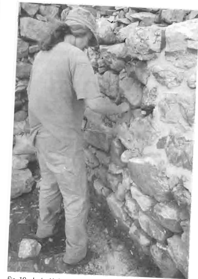
Fig. 19 - Janka Verhey working on the consolidation of the walls.
