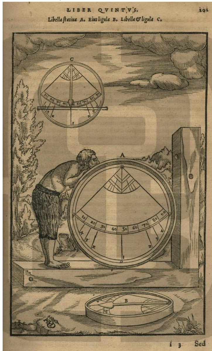
Illustration 15: Illustration of a Mason's Level in the Latin De re metallica Specimen Used by Schall von Bell for the Translation
