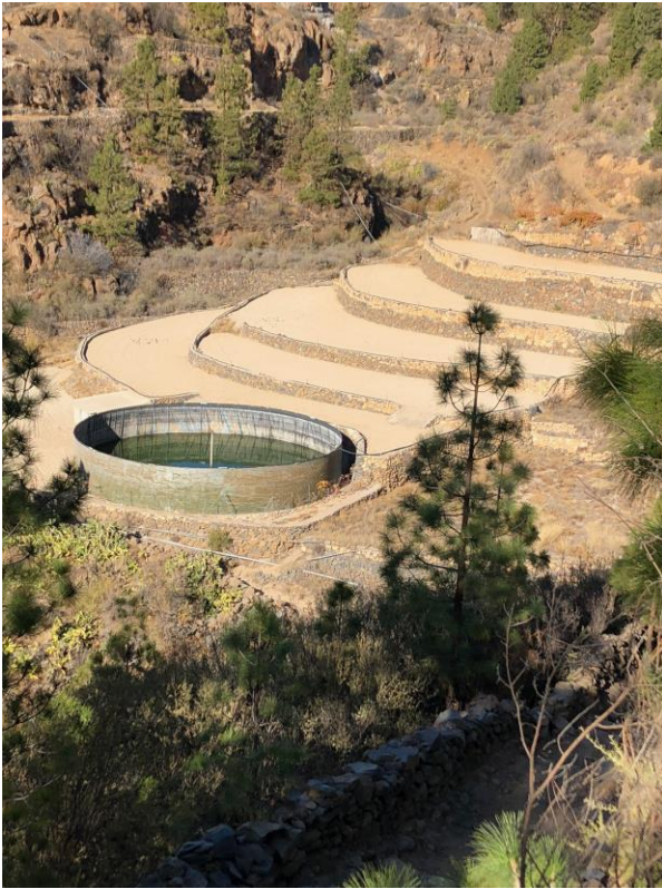
Terraced rain water collection systems for agriculture in Vilaflor on the Canary Island of Tenerife. Photo: Laura Dierksmeier
