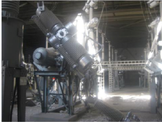
Okuma line 1L (O-81) Circuit Breaker damaged
