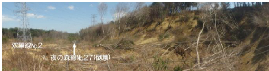
Overview of landslide
