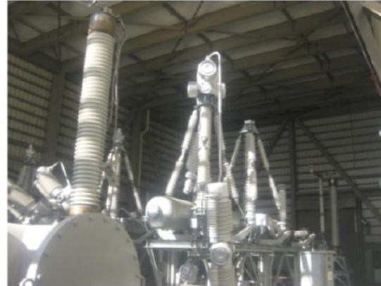
Okuma line 2L (O-81) Circuit Breaker damaged
