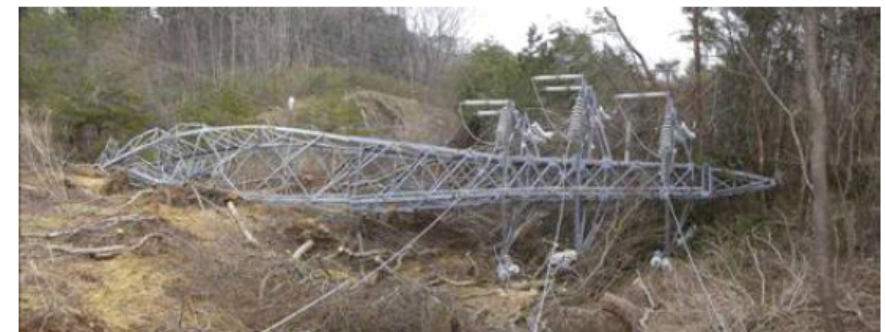
Collapsed tower
